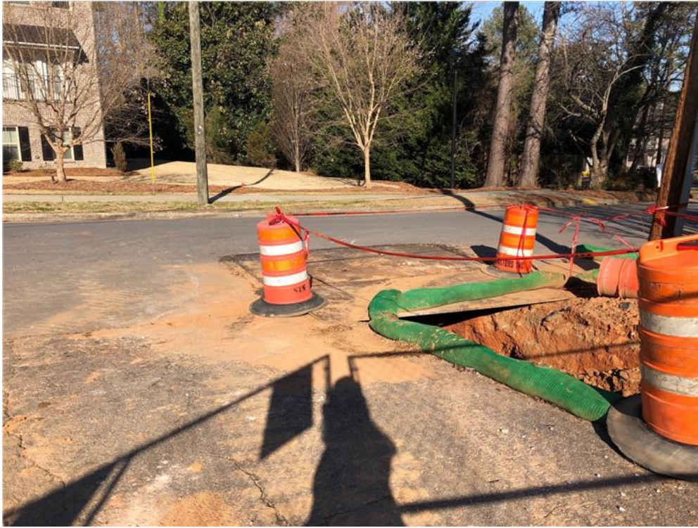
Remove sediment end of each work day
